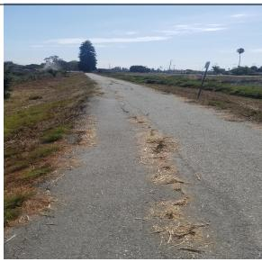
Inspect ID: PJRU\_2019\_a\_0006 Title: USACE\_CESPN\_PJRU\_2019\_a\_0006\_2.jpg Rated Item: 9. Cracking Caption: Rating: Minimally Acceptable; Remarks: Longitudinal cracking observed along the crest of the levee prism.; Action: Cracks should be sealed; Station\_1: 30+00
