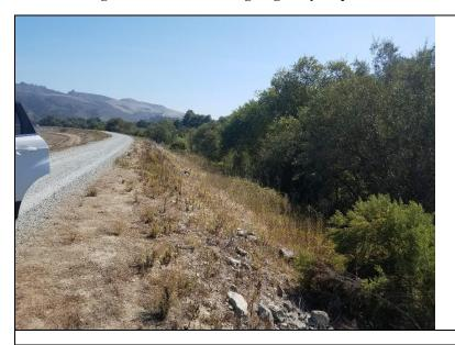
Inspect ID: PJRU\_2019\_a\_0019 Title: USACE\_CESPN\_PJRU\_2019\_a\_0019\_1.jpg Rated Item: 12. Riprap Revetments & Bank Protection Caption: Rating: Minimally Acceptable; Remarks: Vegetation growing through the riprap on the waterside slope of the levee prism.; Action: Remove vegetation growth and restore any displaced riprap.; Station 1: 565+00
