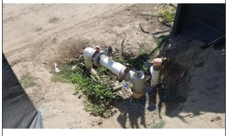
Inspect ID: PJRU\_2019\_a\_0004 Title: USACE\_CESPN\_PJRU\_2019\_a\_0004\_1.jpg Rated Item: 3. Encroachments Caption: Rating: Unacceptable; Remarks: Unauthorized drainage pipes encroaching into the landside toe of the levee prism.; Action: Encroachment should be permitted or otherwise removed.; Station 1: 47+00
