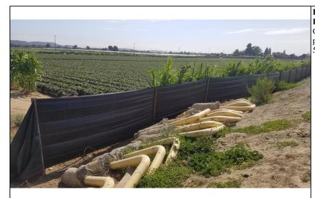
Inspect ID: PJRU\_2019\_a\_0003 Title: USACE\_CESPN\_PJRU\_2019\_a\_0003\_1.jpg Rated Item: 3. Encroachments Caption: Rating: Minimally Acceptable; Remarks: Construction materials and debris observed encroaching on the landside toe of the levee prism.; Action: Encroachments should be permitted or otherwise removed.; Station\_1: 54+00
