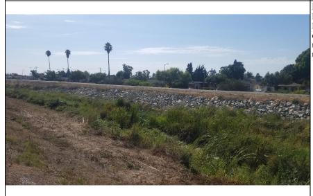
Inspect ID: PJRU\_2019\_a\_0007 Title: USACE\_CESPN\_PJRU\_2019\_a\_0007\_1.jpg Rated Item: 2. Shoaling (sediment deposition) Caption: Rating: Unacceptable; Remarks: Dense vegetation and shoaling approximately 1000 ft long observed in the channel.; Action: A Hydrologic and Hydraulic analysis should be performed to confirm the capacity of the channel. The shoal should be removed absent analysis demonstrating the hydraulic capacity is otherwise maintained.; Station 1: 27+00
