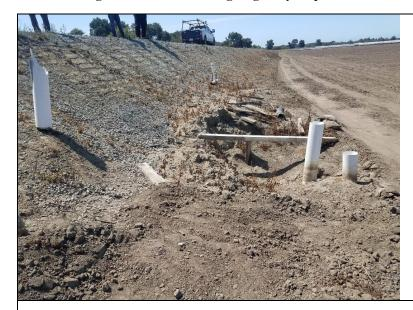
Inspect ID: PJRU\_2019\_a\_0010 Title: USACE\_CESPN\_PJRU\_2019\_a\_0010\_1.jpg Rated Item: 3. Encroachments Caption: Rating: Unacceptable; Remarks: Unauthorized excavation observed at the toe of the landside slope.; Action: Recommend a section 408 modification request be submitted, or the site be restored to as-built conditions and the slope be restored to the lines and grades in the O&M manual.; Station\_1: 363+00
