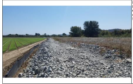
Inspect ID: PJRU\_2019\_a\_0013 Title: USACE\_CESPN\_PJRU\_2019\_a\_0013\_1.jpg Rated Item: 3. Encroachments Caption: Rating: Minimally Acceptable; Remarks: Gravel deposited at the toe of the landside slope.; Action: Recommend a section 408 modification request be submitted, or the area should be restored to as-built conditions.; Station 1: 410+00
