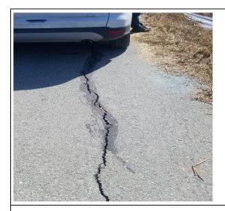
Inspect ID: PJRU\_2019\_a\_0006 Title: USACE\_CESPN\_PJRU\_2019\_a\_0006\_1.jpg Rated Item: 9. Cracking Caption: Rating: Minimally Acceptable; Remarks: Longitudinal cracking observed along the crest of the levee prism.; Action: Cracks should be sealed; Station 1: 30+00
