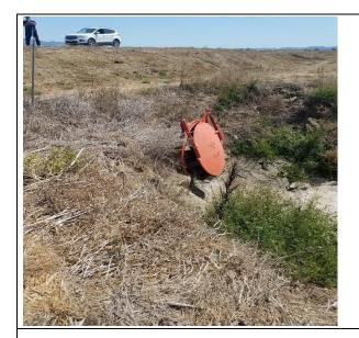
Inspect ID: PJRU\_2019\_a\_0012 Title: USACE\_CESPN\_PJRU\_2019\_a\_0012\_1.jpg Rated Item: 11. Flap Gates/ Flap Valves/ Pinch Valves Caption: Rating: Minimally Acceptable; Remarks: Flap gate blocked by debris and vegetation growth.; Action: Debris should be removed, and flap gate operational status should be confirmed.; Station\_1: 392+00
