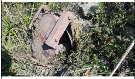
**Inspect ID:** PJRU\_2019\_a\_0005 **Title:** USACE\_CESPN\_PJRU\_2019\_a\_0005\_2.jpg **Rated Item:** 11. Flap Gates/ Flap Valves/ Pinch Valves **Caption:** Rating: Minimally Acceptable; Remarks: Interior drainage flap gate blocked by sediment and vegetation.; Action: Remove obstruction from flap gate outflow path and confirm the flap gate is functional.; Station 1: 34+00
